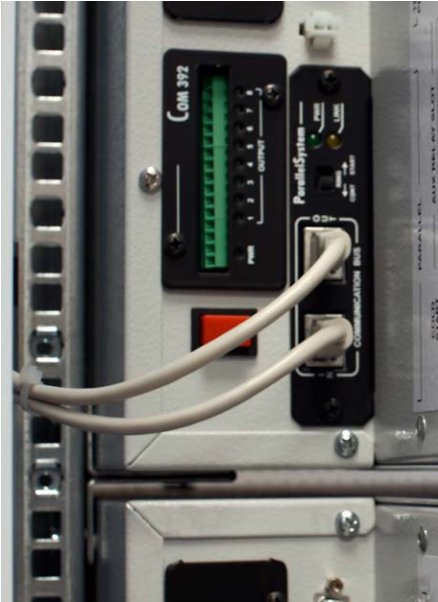
Parallel configuration and programmable relay contacts board
